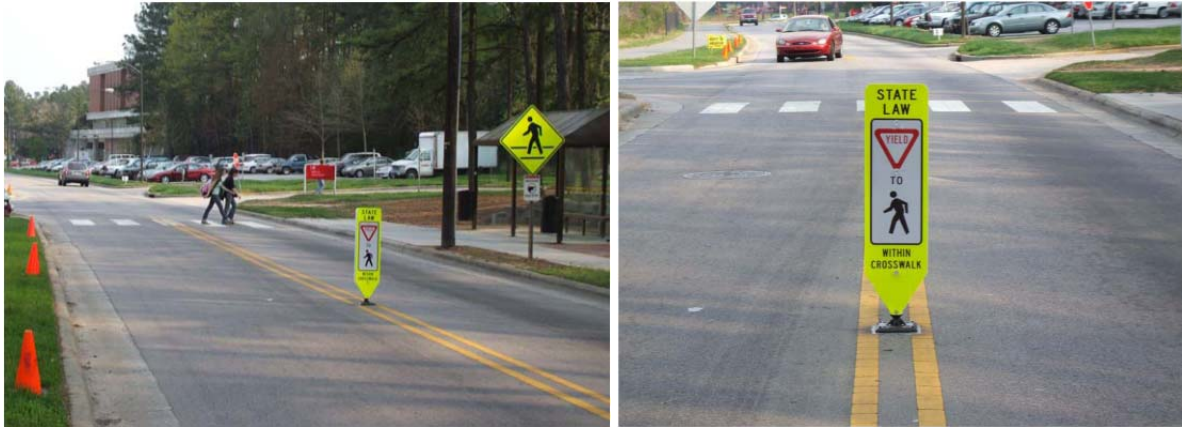
Image 1: example of a pedestrian safety installation, alerting drivers of the upcoming crosswalk.
