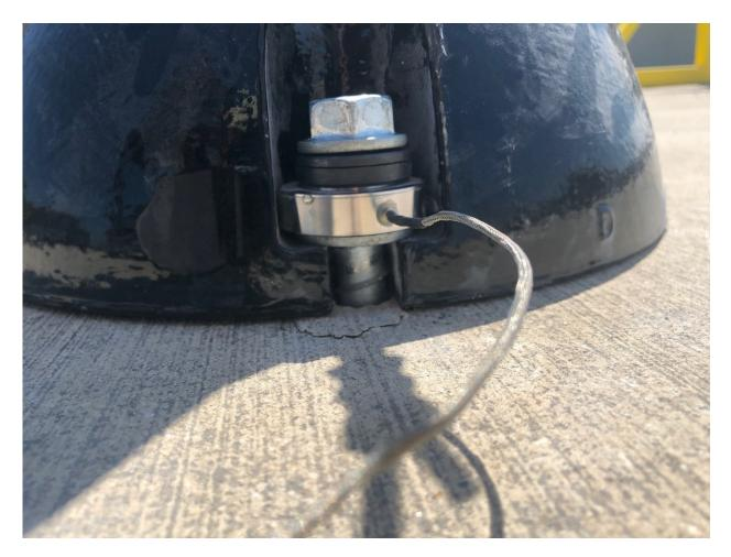
Figure 4 - Spalled Concrete
