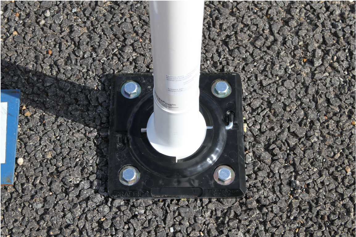
Figure B4. Delineators Attached to Asphalt prior to Testing.
