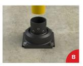
Insert the pipe into the adapter.
