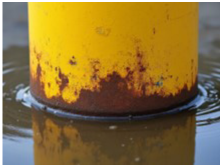
Figure 6 - Bollard Corrosion
