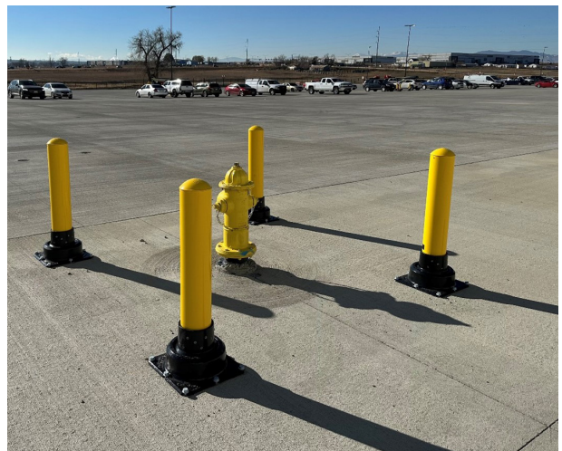
Figure 4 - SlowStop Fire Hydrant Protection
