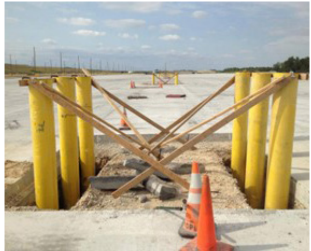
Figure 2 - Greenfield Bollard Installation
