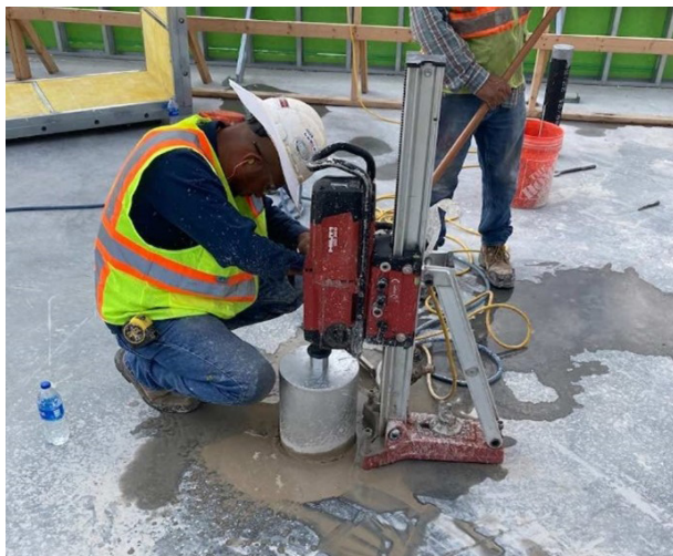
Figure 3 - Core Drilling
