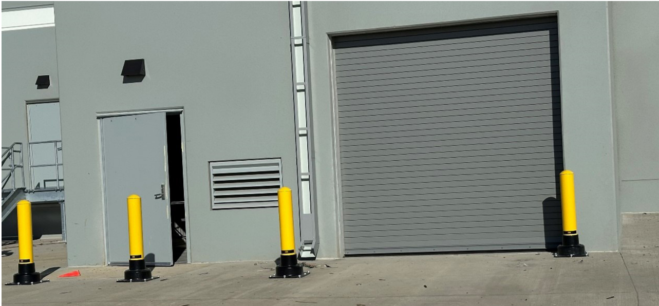
Figure 1 - Surface Mount Rebounding Bollards
